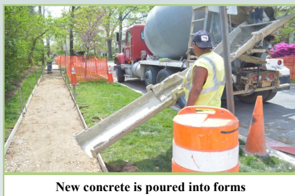
New concrete is poured into forms
